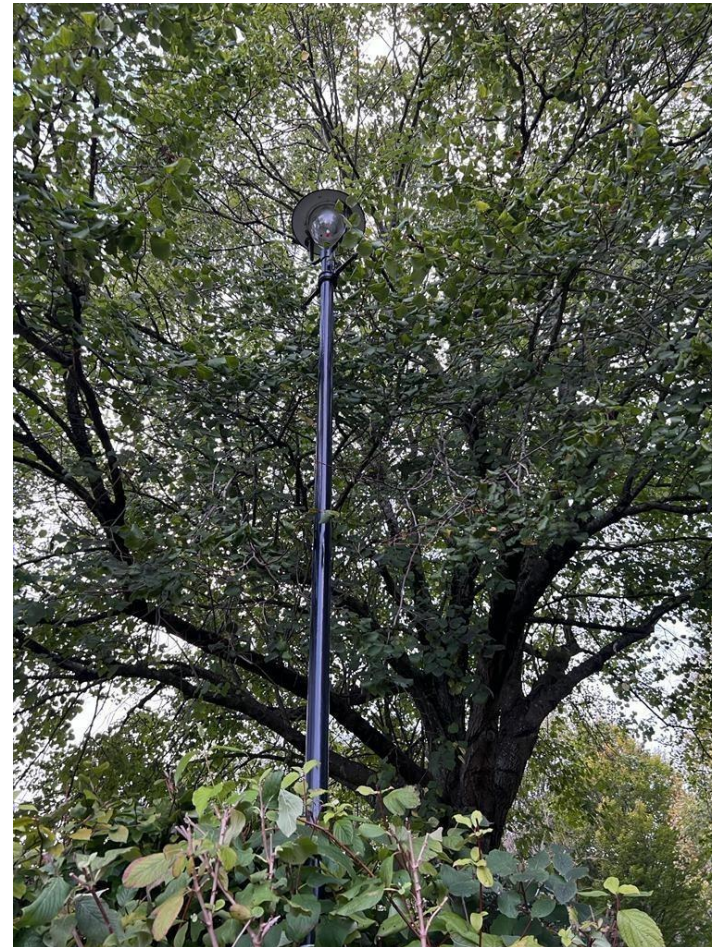
Photo 30 – Lime tree (T28) branches impeding street light
