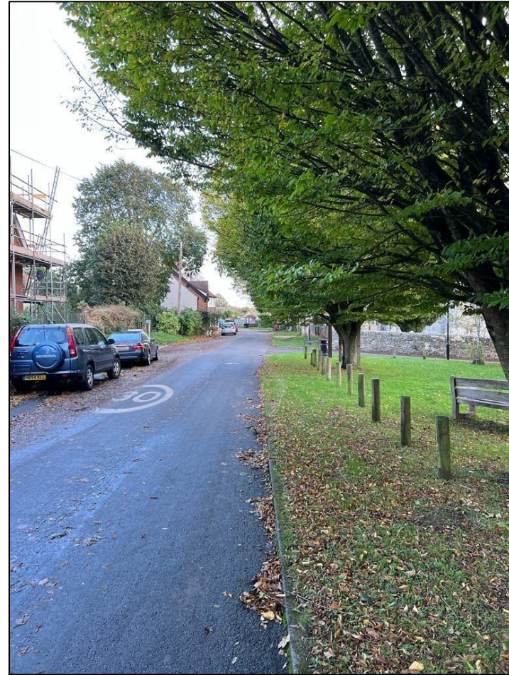
Photo 18 _ Branches impinging the highway along Dorchester Road
