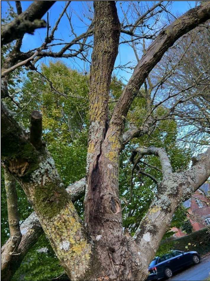
Photo 23 _ Failed union on potentially dead tree (T12)
