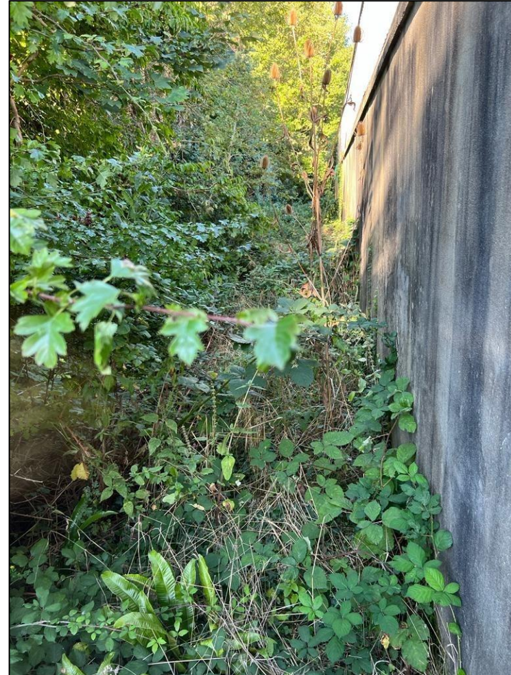
Photo 10 – Vegetation next to retaining wall (G3)
